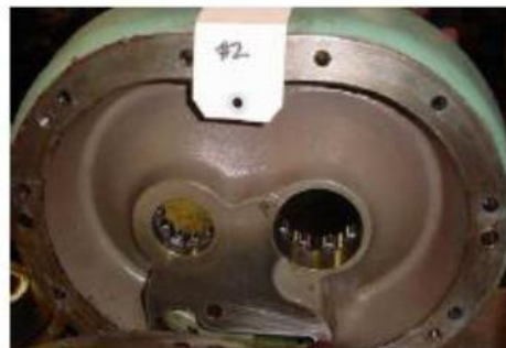
Inlet Rotor Average Varnish: 9.8 Sludge: 9.5
