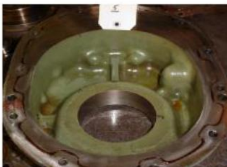
Gear Case Front Housing Varnish: 9.8 Sludge: 9.5
